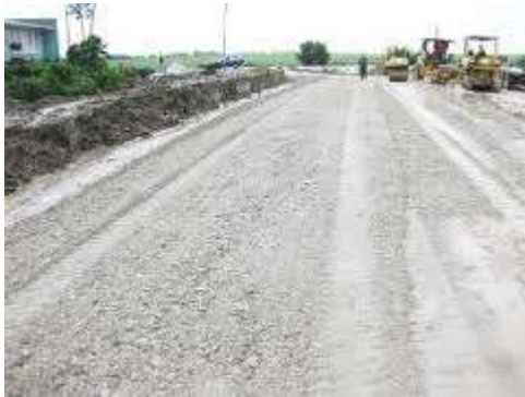
Road crusher run
