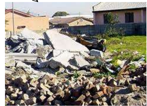
Rubble and soil waste
